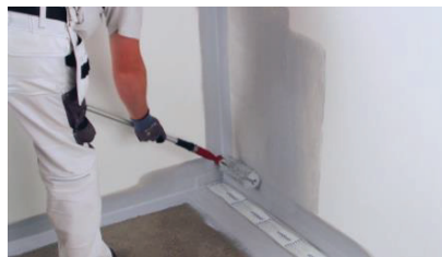
Apply first coat of LIP VS30 to all areas shown below using a roller.
