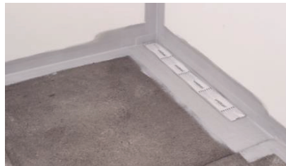
Apply another coat of VS30 over reinforcement tape.
